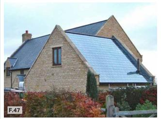
**Figure 47:** Solar panels should be integrated into the design of buildings from the outset. This example of a new home in a Conservation Area shows how the panels can mimic the appearance of traditional slate roofs.
