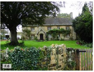
Figure 06: Example of a coursed square rubble facade.
