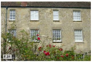
**Figure 31:** Well-proportioned and placed sash windows that are slightly setback into the facade and feature glazing bars.
